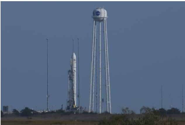
Left: The 139 feet tall Antares 230+ rocket is vertical on the Mid-Atlantic Regional Spaceport's (MARS) launch pad OA. This launch pad is used for liquid fueled medium class orbital rockets. Adjacent to the rocket is the 307 feet tall water tower used for water deluge and acoustical suppression.
